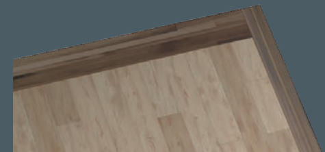
LVL & hardwood rigid outer frame.
